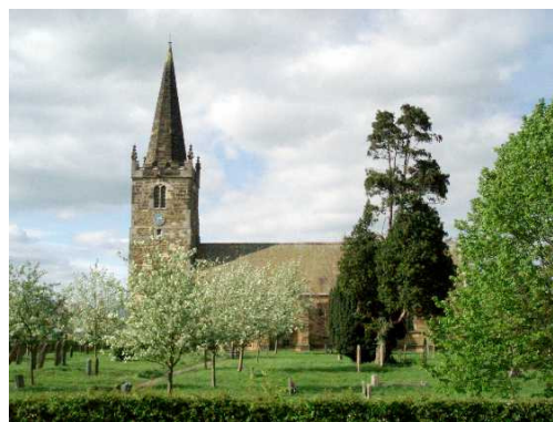
St Catherine's Church, looking north
