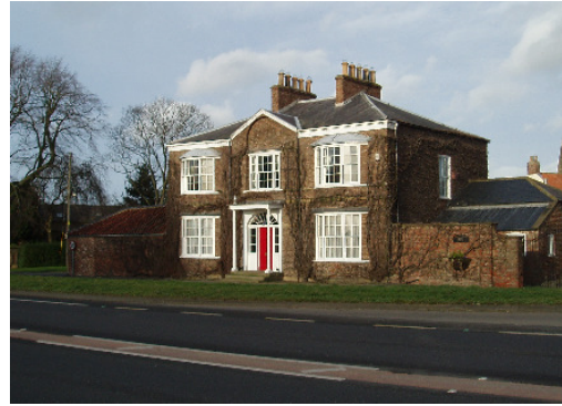
Barmby Moor House, from the south east
